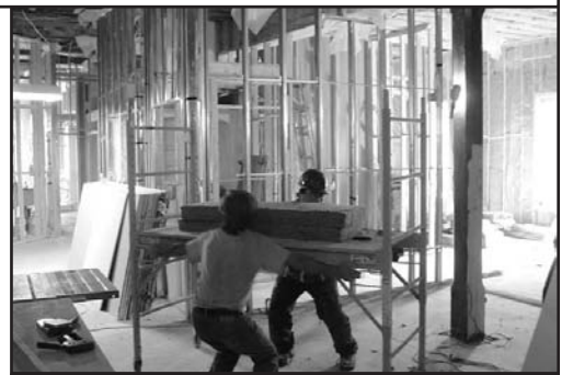
Workers hired through a Job Creation Partnership work on drywalling and insulating the apartments on the second floor of 66 Queen St. S.
