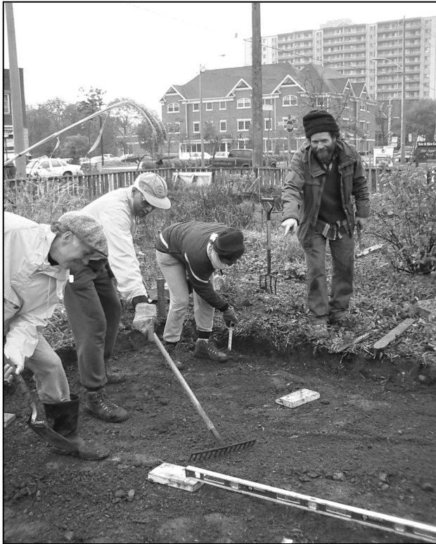
Above: Digging out & levelling the foundation area.
