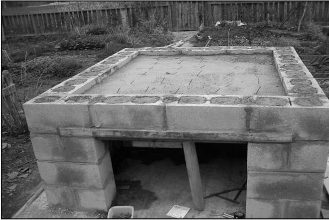
Below: Rebar bars grooved into blocks. Wood form around rebar keeps the oven slab apart from the block wall.
