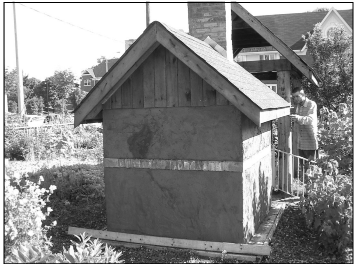
Above: A back view of the entire oven, with roof and front shelter. Notice the cement parging on walls and sides which has covered the concrete block wall.
