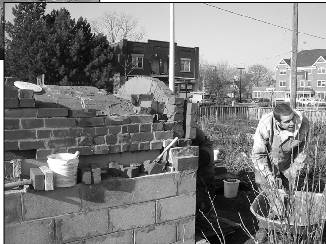
Below: Mixing mortar in small batches in the wheelbarrow.
