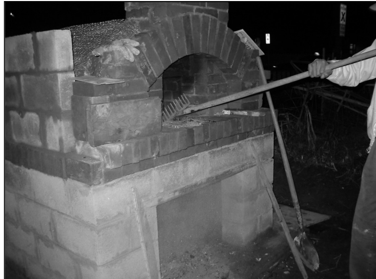
Below: Raking ashes through the ash slot. A simple garden rake and wet mop are useful tools. A metal bucket goes underneath ash slot, in front of wood storage vault, to catch the embers/ashes.
