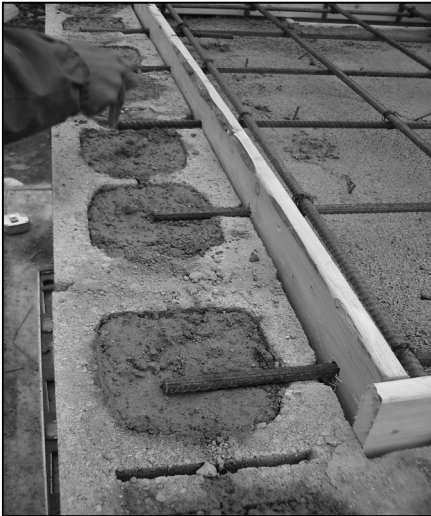
Below: Rebar bars grooved into blocks. Wood form around rebar keeps the oven slab apart from the block wall.
