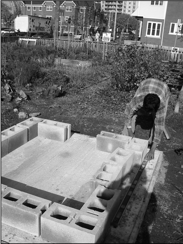
Above: After the wall dimensions have been marked out, it's time to lay the concrete blocks. They are carefully positioned onto mortar which has been prepared.
