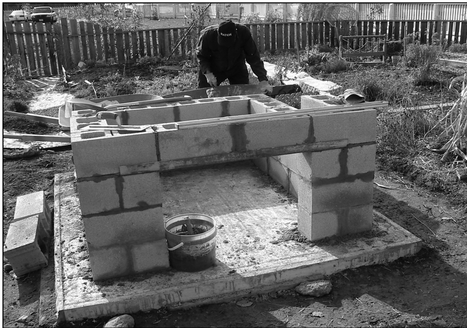
Below: Second view of block walls. Notice the 4-foot level - it is important to always check the levels at each stage!
