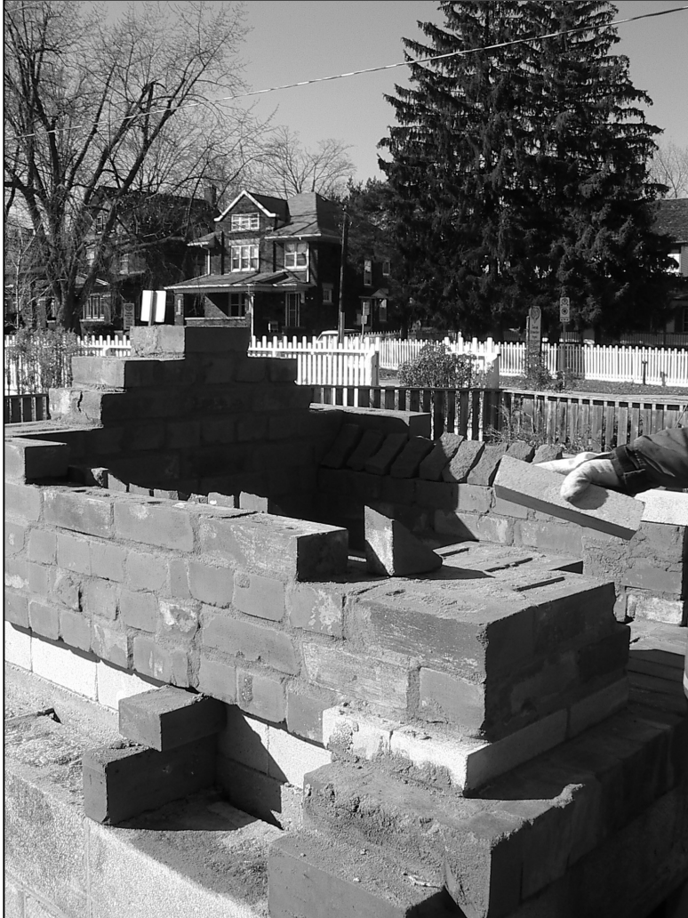
Left: Height of the oven wall – note gable, doorway & door height.
