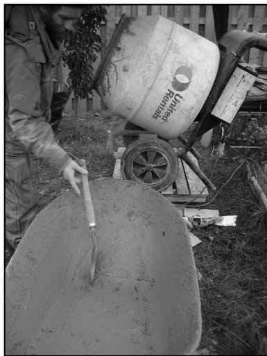
Left: Third, mix concrete by electric mixer or by hand. Remember to wet the inside of the electric mixer to prevent cement dust flying when the motor starts up! 3-4 bags fit per mixer load. Add more water as necessary to make it a workable consistency. A group of 4-5 people is good to have for a speedy flow of materials.
