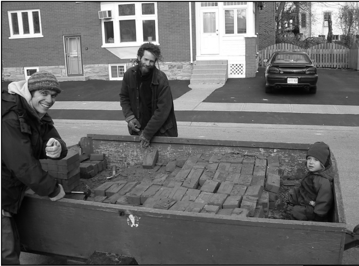
Left: Cleaning and chiseling old mortar off the reclaimed bricks.
