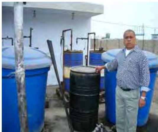
Mr A Jacobo with the current biodiesel reactor (Photo: Practical Action)
