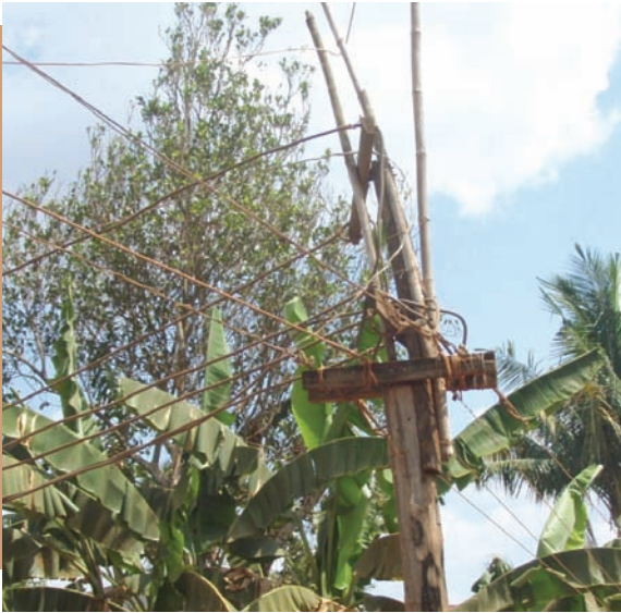
Electricity distribution to 80 consumers
